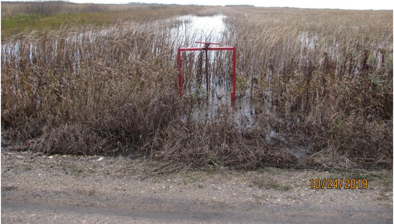
Lat 8 SD 72 – Existing Mel Wang Pipe looking to the north
