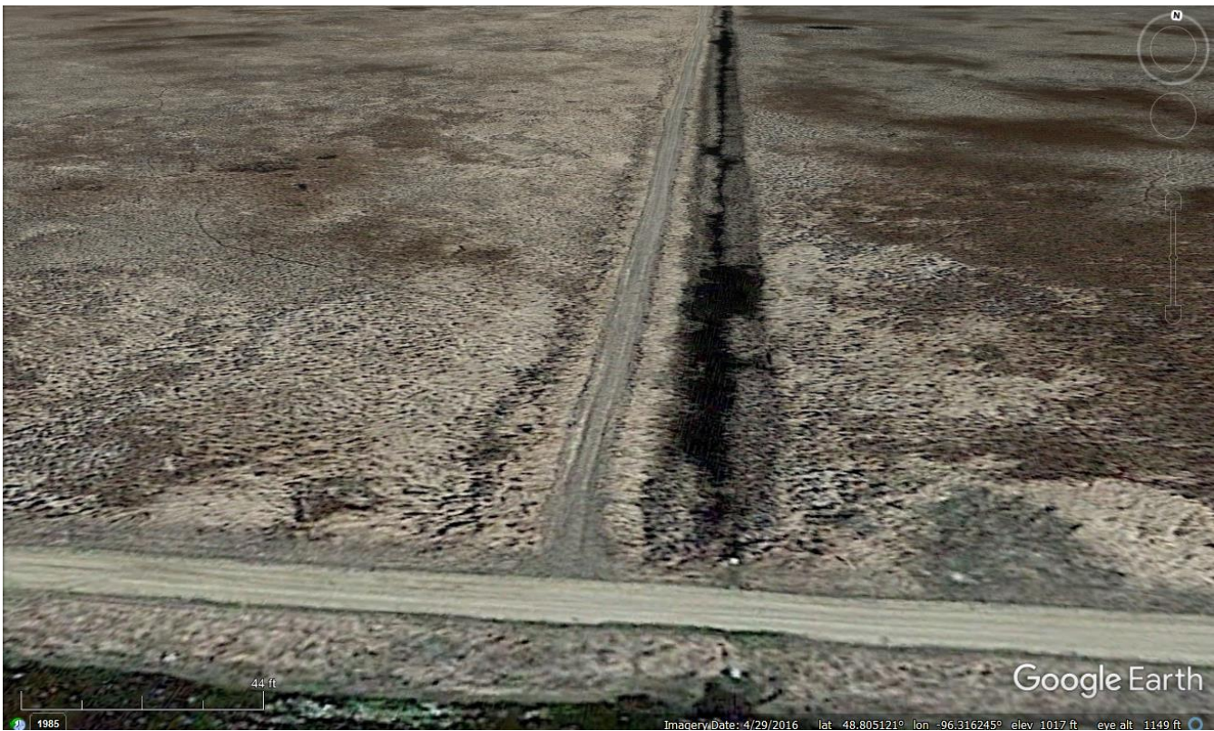
Lat 8 SD 72 – Existing Mel Wang Pipe looking to the north
